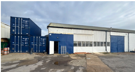
Brewery and taproom - work in progress
